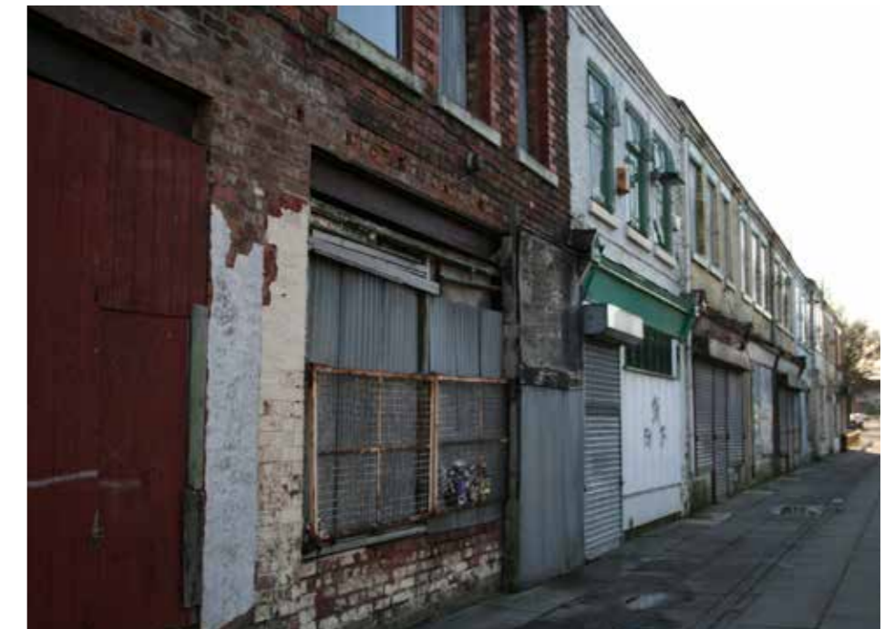
Photo 55: Vacant shops that front onto A552
