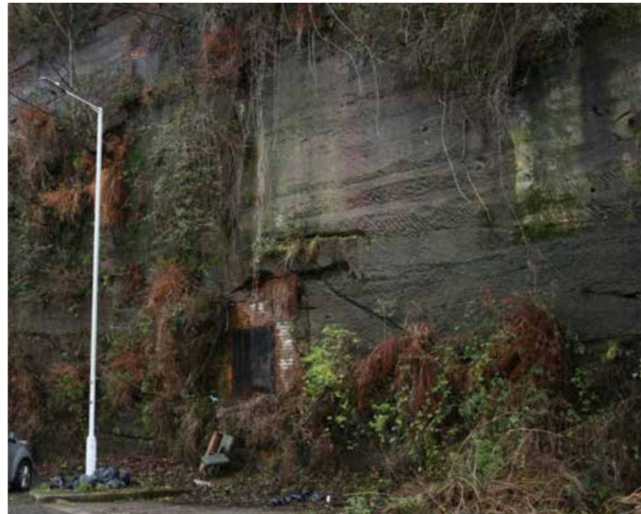
Photo 8: Tranmere Tunnels entrance at Holborn Square
