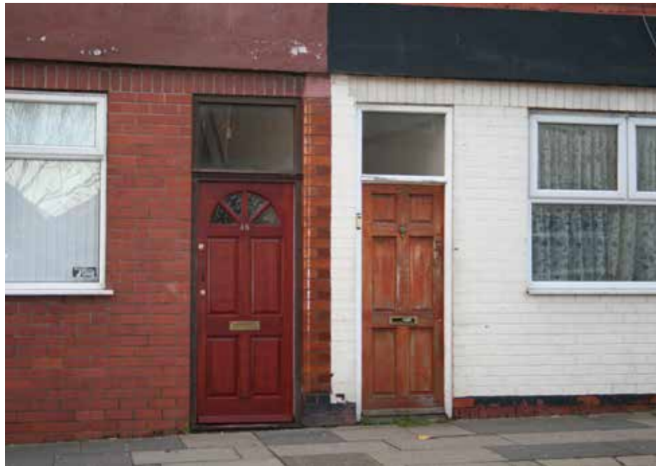
Photo 38: Example of glazed tiles, Derby Road
