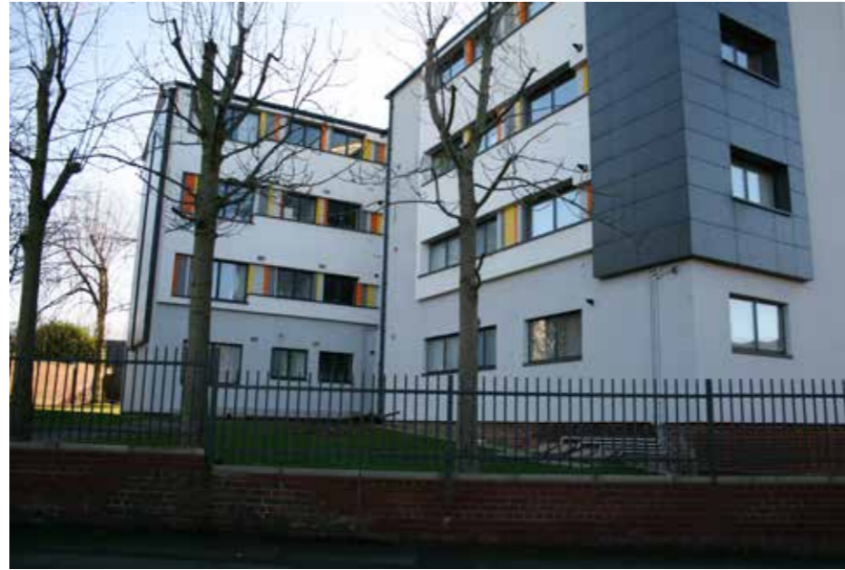
Photo 42: Example of modern flats, Quarry Bank
