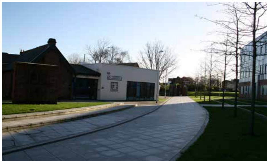
Photo 21: Public Realm adjacent to St Catherine's Health Centre
