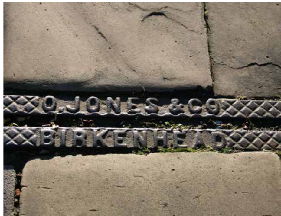
Photo 54: Example of cast iron detailing, Whalley Road
