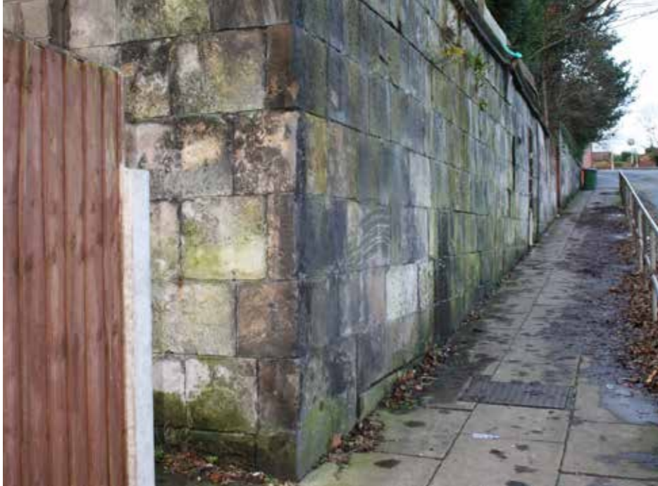
Photo 26: Example of stone retaining walls and guardrails to slopes, Holt Hill
