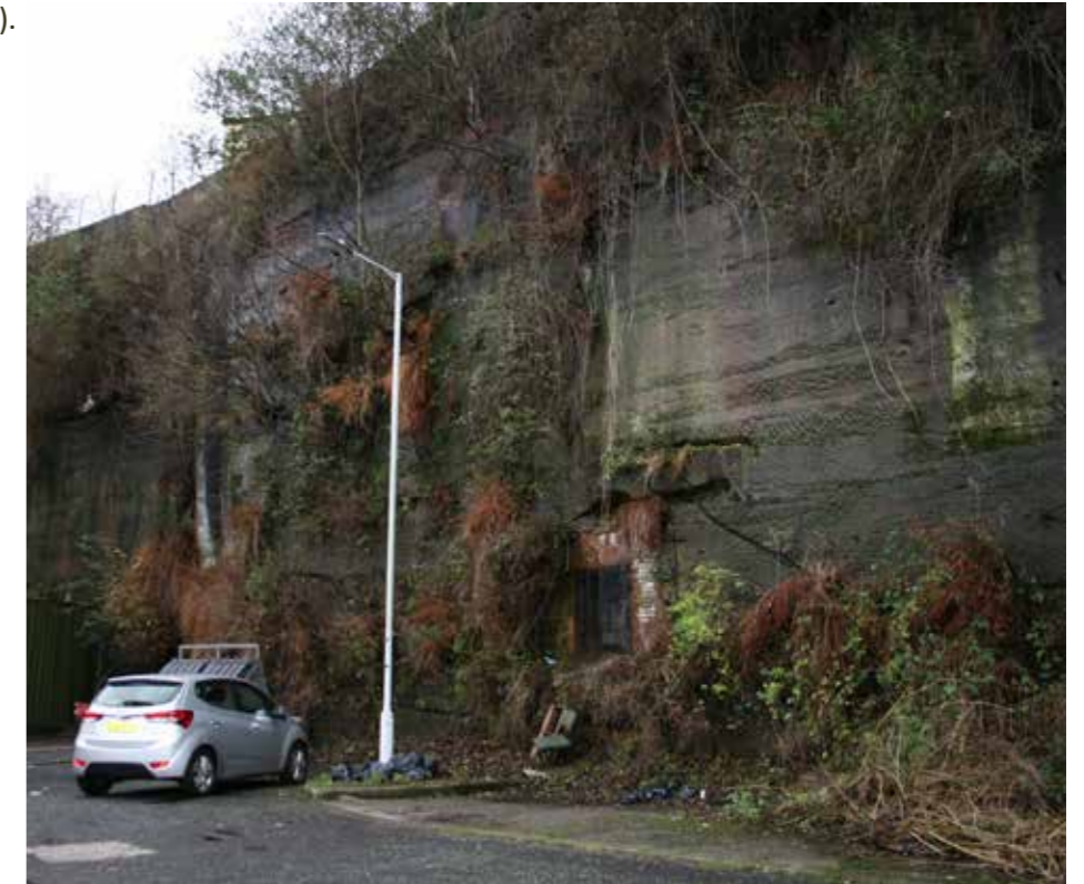
Photo 24: Tranmere Tunnels entrance, Holborn Square
