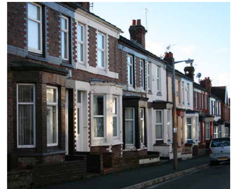
Photo 50: Example of architectural detailing to frontages
